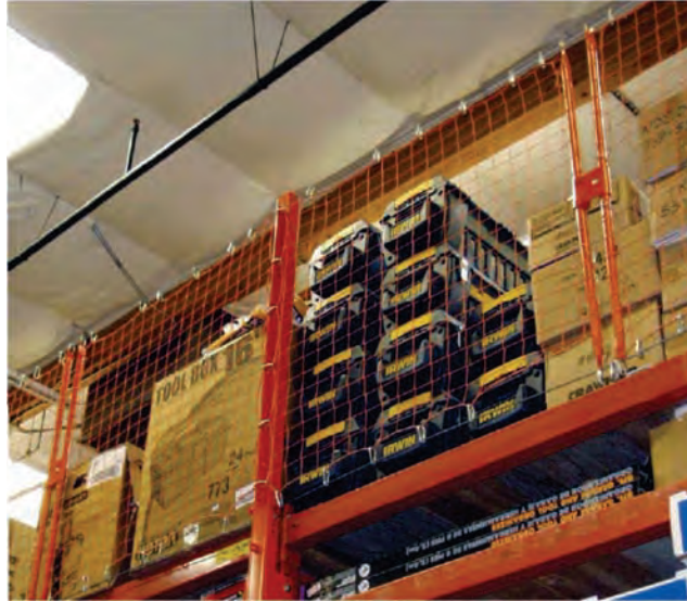
Figure C15.5-1 Merchandise restrained by netting.
