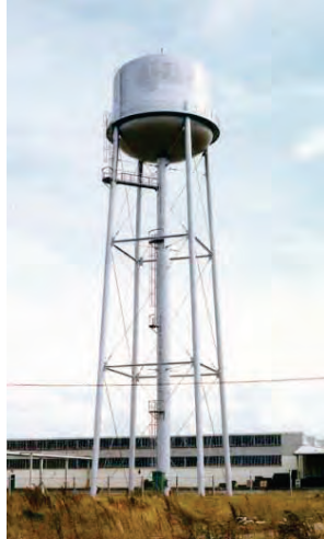
Figure C15.7-1 Multi-leg braced steel tank.
