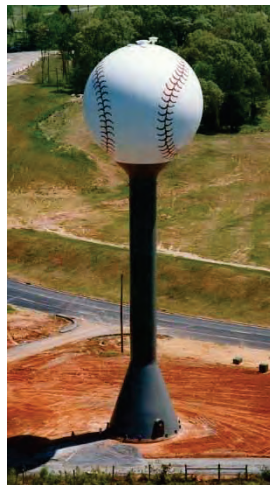
Figure C15.7-2 Small-diameter single-pedestal steel tank.
