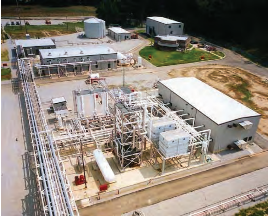
Figure C15.1-2 Steel pipe rack.
