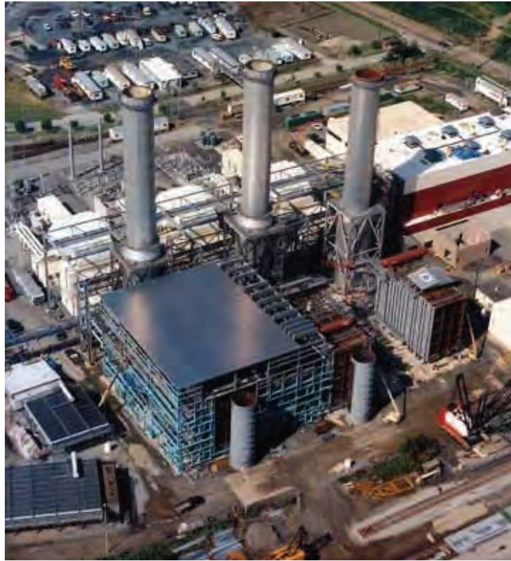
Figure C15.1-3 Heat recovery steam generators.
