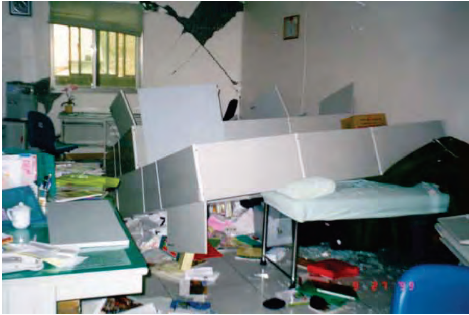
Figure C13.1-5 Toppled storage cabinets.
