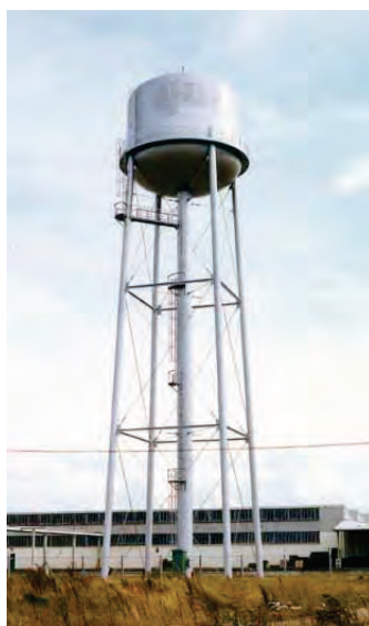
Figure C15.1-1 Steel multi-legged water tower.
